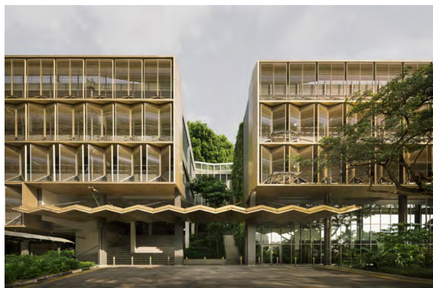
The extended west façade of the Equatorial School at NUS, Singapore, is designed as an envelope that engages with the tropical climate, screening the building from heat gain by creating a deep veil | Image by Finbarr Fallon; Courtesy of Erik L'Heureux, FAIA; Campus Design Innovations Group, National University of Singapore; and DP Green. Source: www.aiany.org
