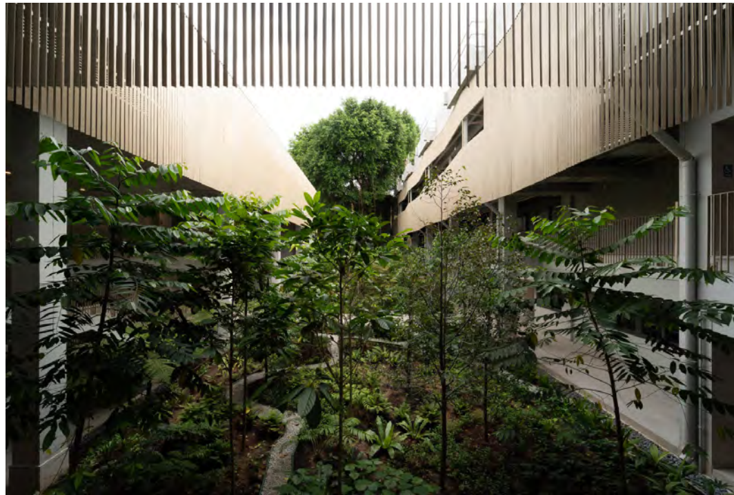
Circulation spaces such as corridors and stairways at the school are entirely naturally ventilated | Image by Finbarr Fallon; Courtesy of Erik L'Heureux, FAIA; Campus Design Innovations Group, National University of Singapore; and DP Green. Source: www.aiany.org
